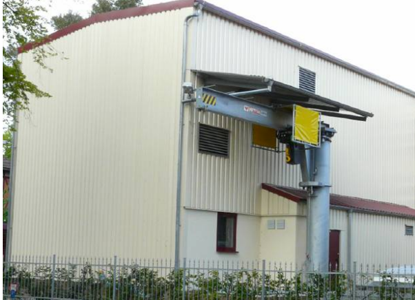
Figure 1: The new Modulator Test Hall
