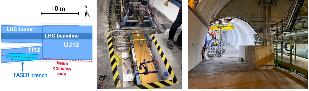
FIG. 5. Map of the TI12 tunnel and UJ12 cavern (left); view of the trench with the FASER \nu emulsion detector installed (center); and available space in the UJ12 tunnel behind FASER (right).
