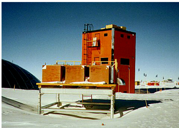
Figure 1: Photo of the three detector tubes in the initial installation of the NM-64 neutron monitors at the South Pole. The neutron monitors are on an elevated platform in insulated, heated boxes. Also shown in the background are the Skylab building (housing the monitor electronics, among others) and part of the iconic Dome (credit: L. Shulman/Bartol).
