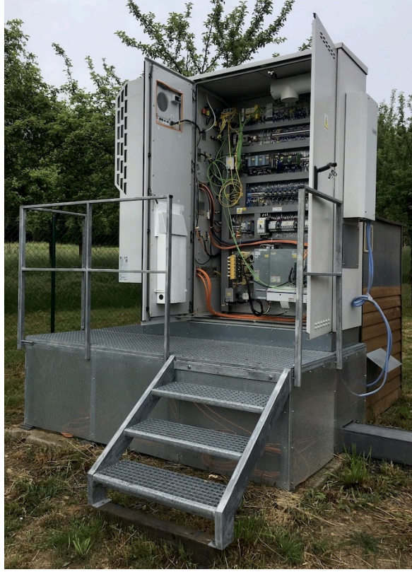
Figure 40. Control cabinet of the prototype telescope.
