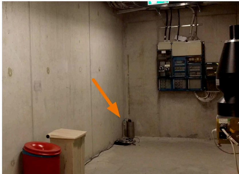
Figure 3.7: The installation site of the seismometer in the 7th underground level of the XSIN building of the European XFEL. (Courtesy: Norbert Meyners)
