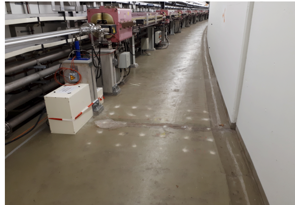
Figure 4: Stabilisation of the transition between two PETRA III tunnel segments.
