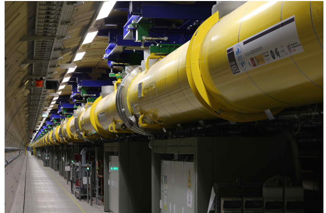
Figure 1: Completed main accelerator in one single tunnel. On top accelerator modules and cable trays. Below RF stations, electronic racks, power and water supply etc.
