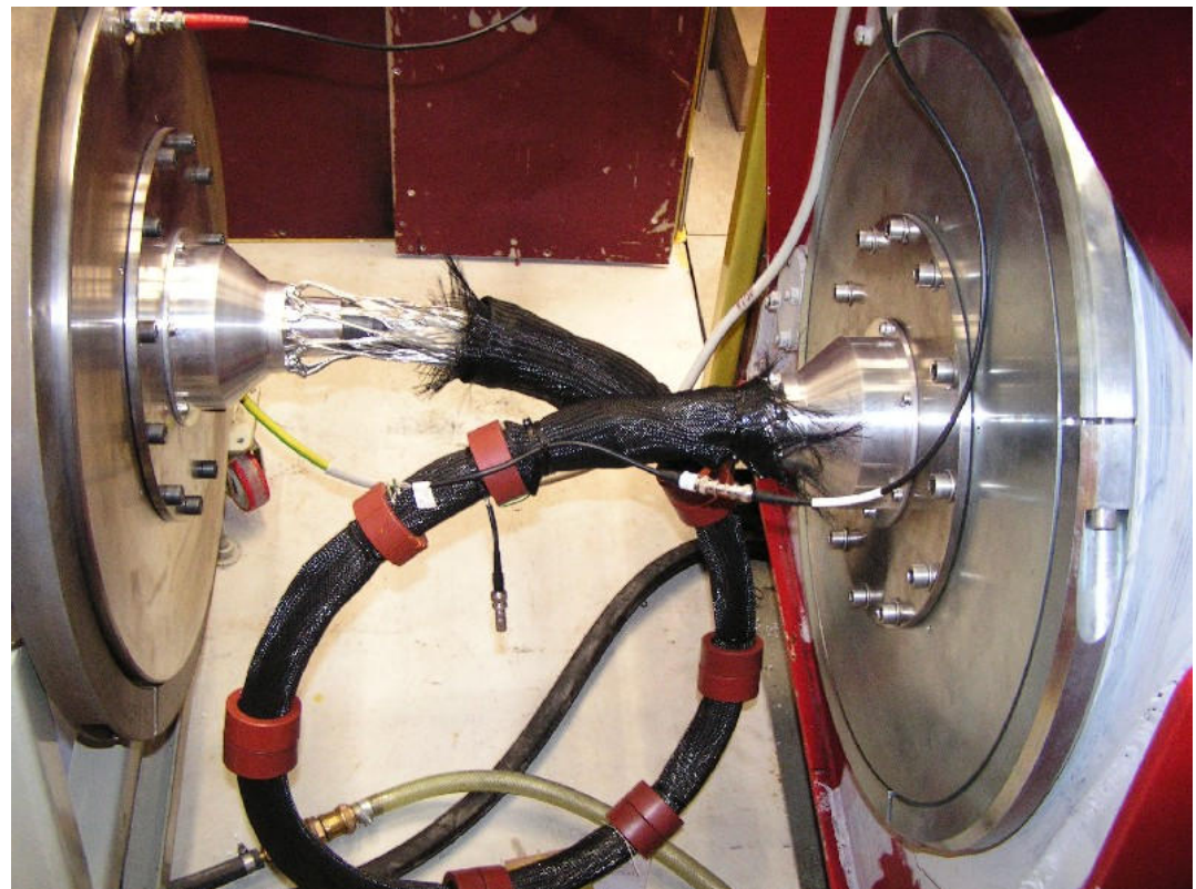
HV cable #2, leakage current ~ 50mA
