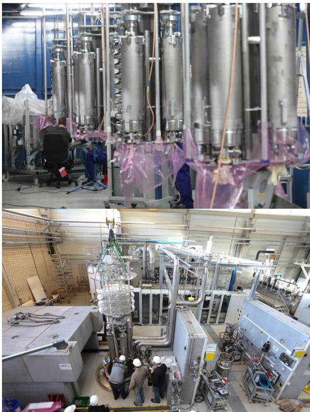
Figure 1: Preparation area for vertical testing (top) and vertical test installations (bottom) at AMTF.
