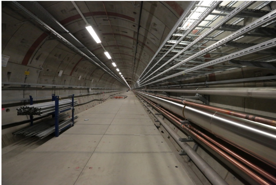
Utilities installed in accelerator tunnel
